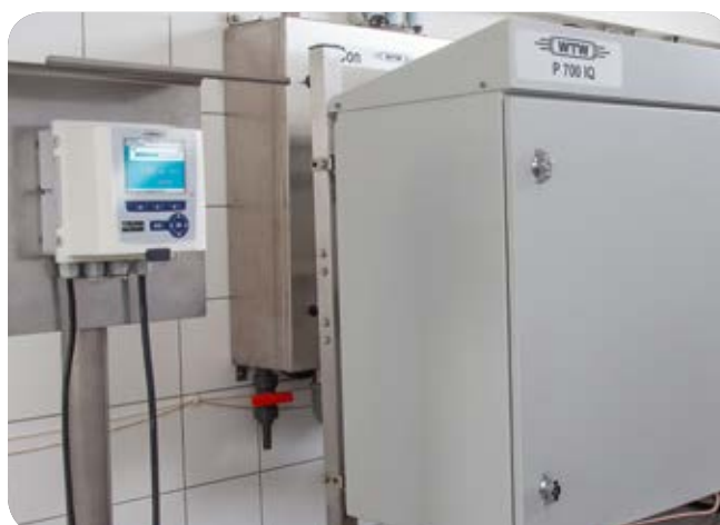
System 282/284 with Phosphate analyzer P 700 IQ
